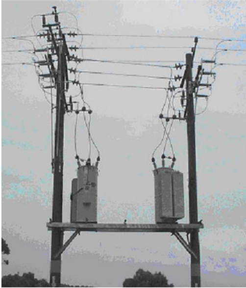
Figure 2 - Typical pole mounted single phase open-delta voltage regulator
