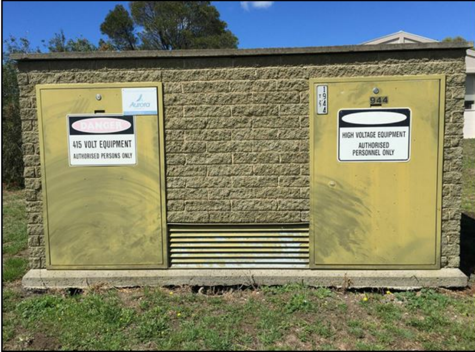
Figure 2 - Kiosk block wall substation
