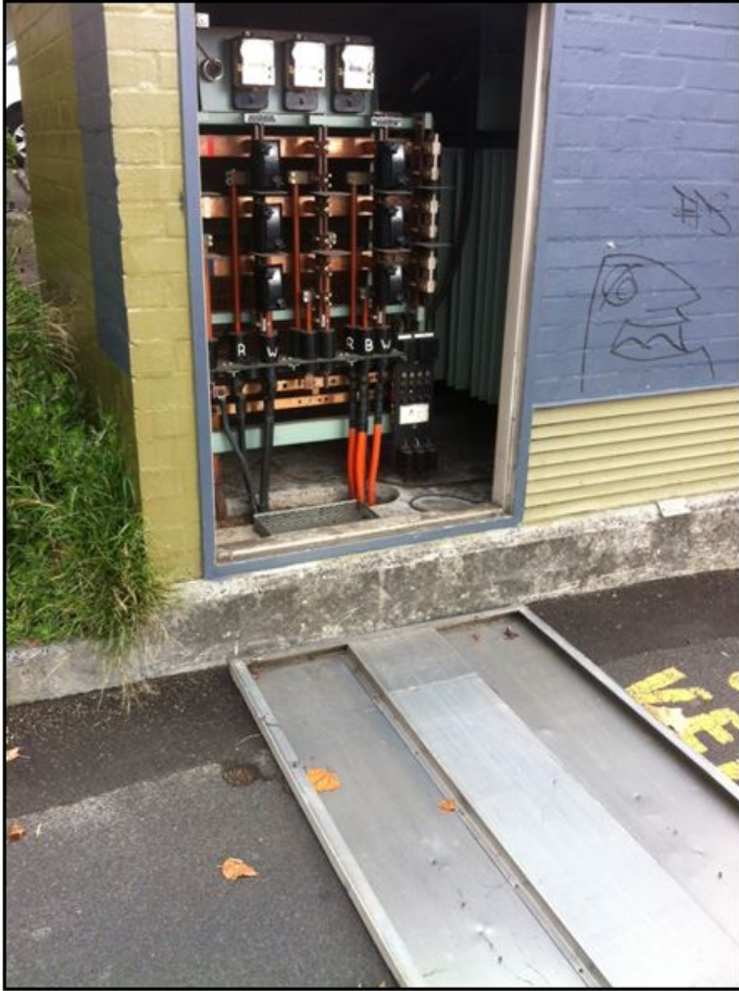
Figure 1 - Door found on ground exposing live front LV board
