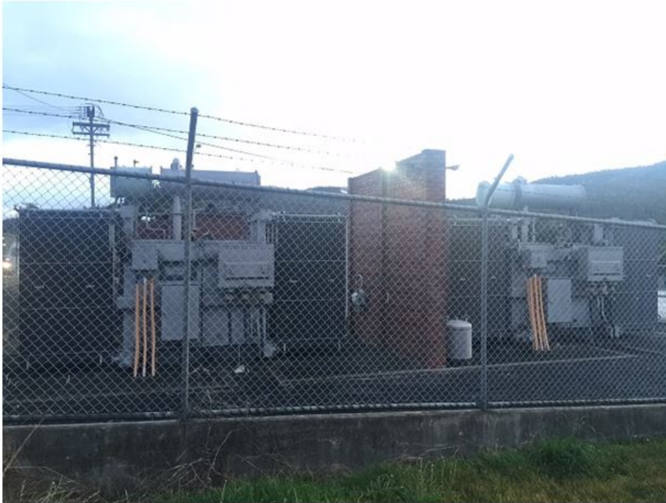
Photo 1 – Bellerive Zone transformers
