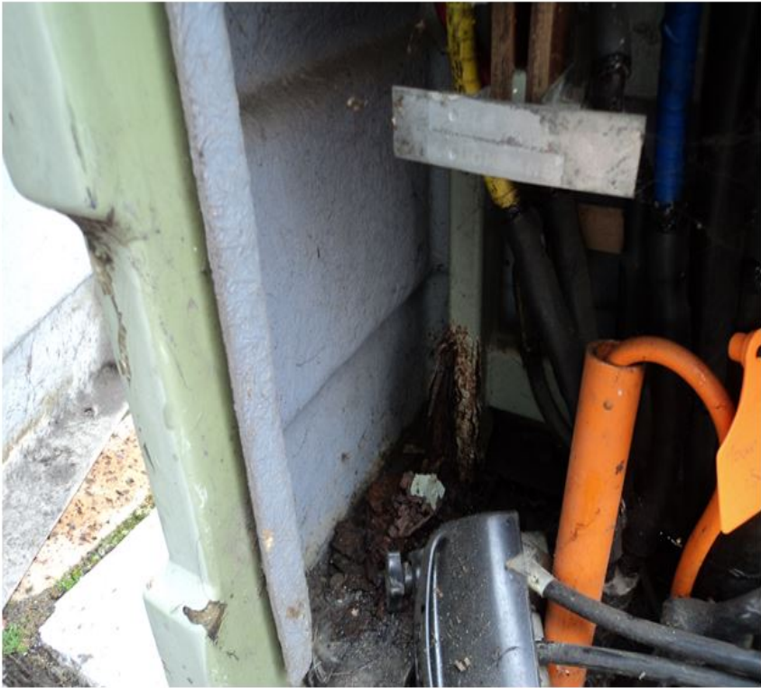
Figure 2 - Low voltage pillar with significant structural corrosion
