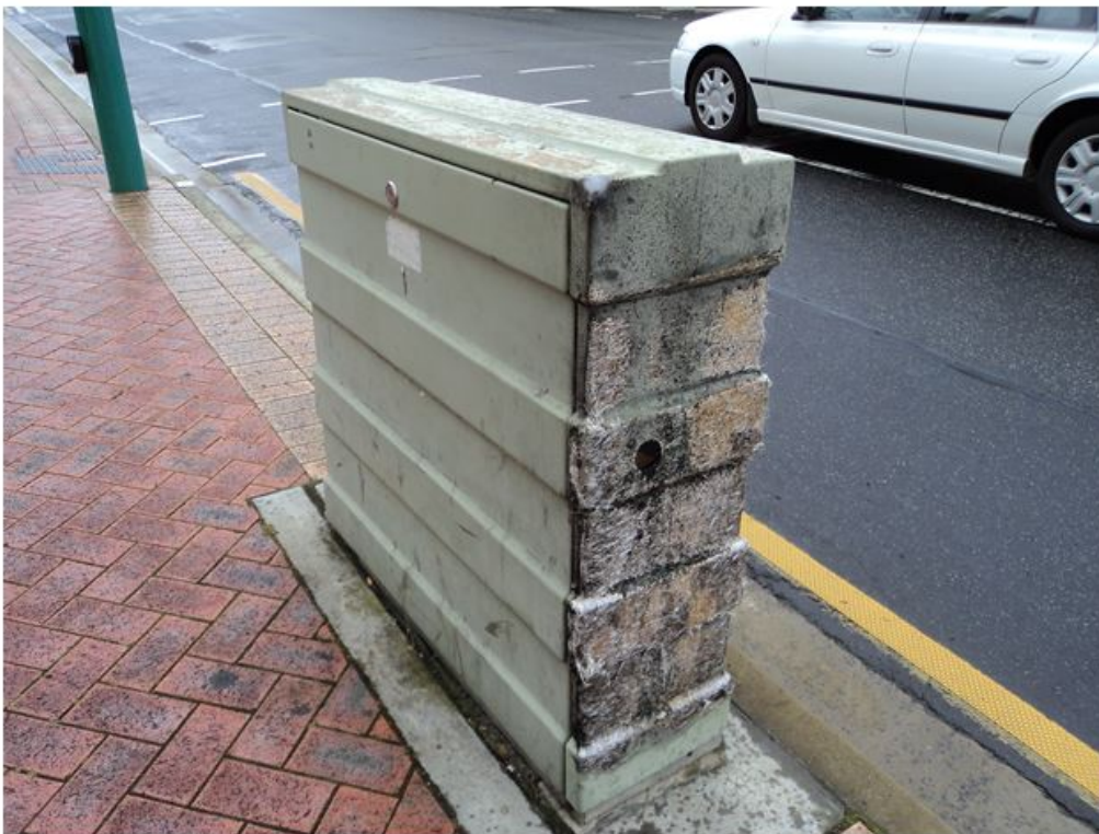
Figure 1 - Fibreglass Pillar with external damage
