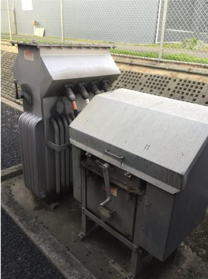
Photo 1 – Bellerive Zone station services transformer and HV switchgear
