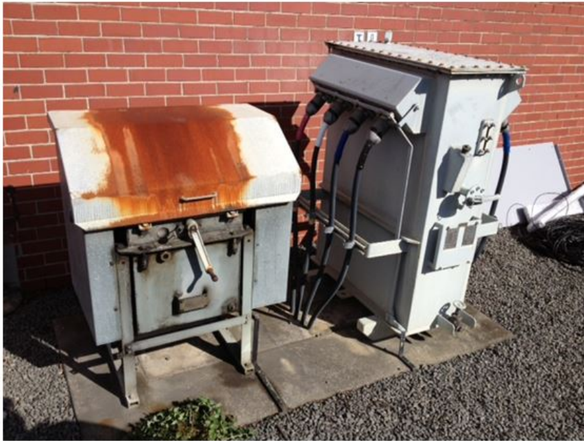
Photo 1 –Services transformer and HV switchgear
