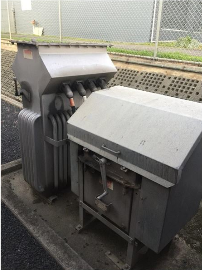
Photo 1 – Station services transformer and HV switchgear
