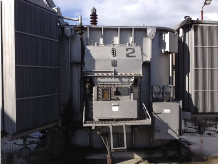
Photo 1 – Derwent Park Zone transformers
