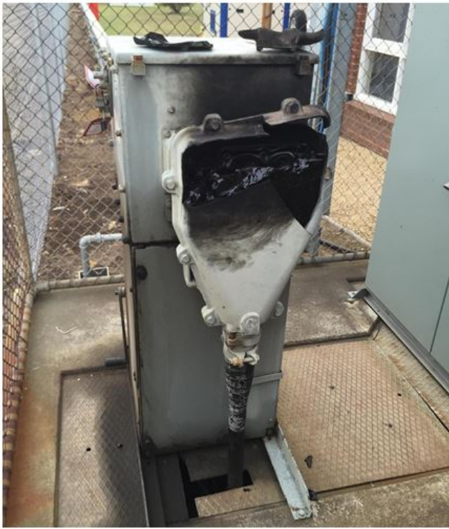
Figure 1 - Recent Reyrolle JKSS switchgear with cast iron pitch filled cable terminations failure - 2014
