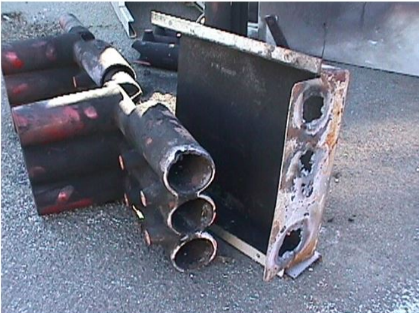
Figure 1 - Epoxy spouts contained inside of RGB switchgear that has failed due to moisture and dust ingress
