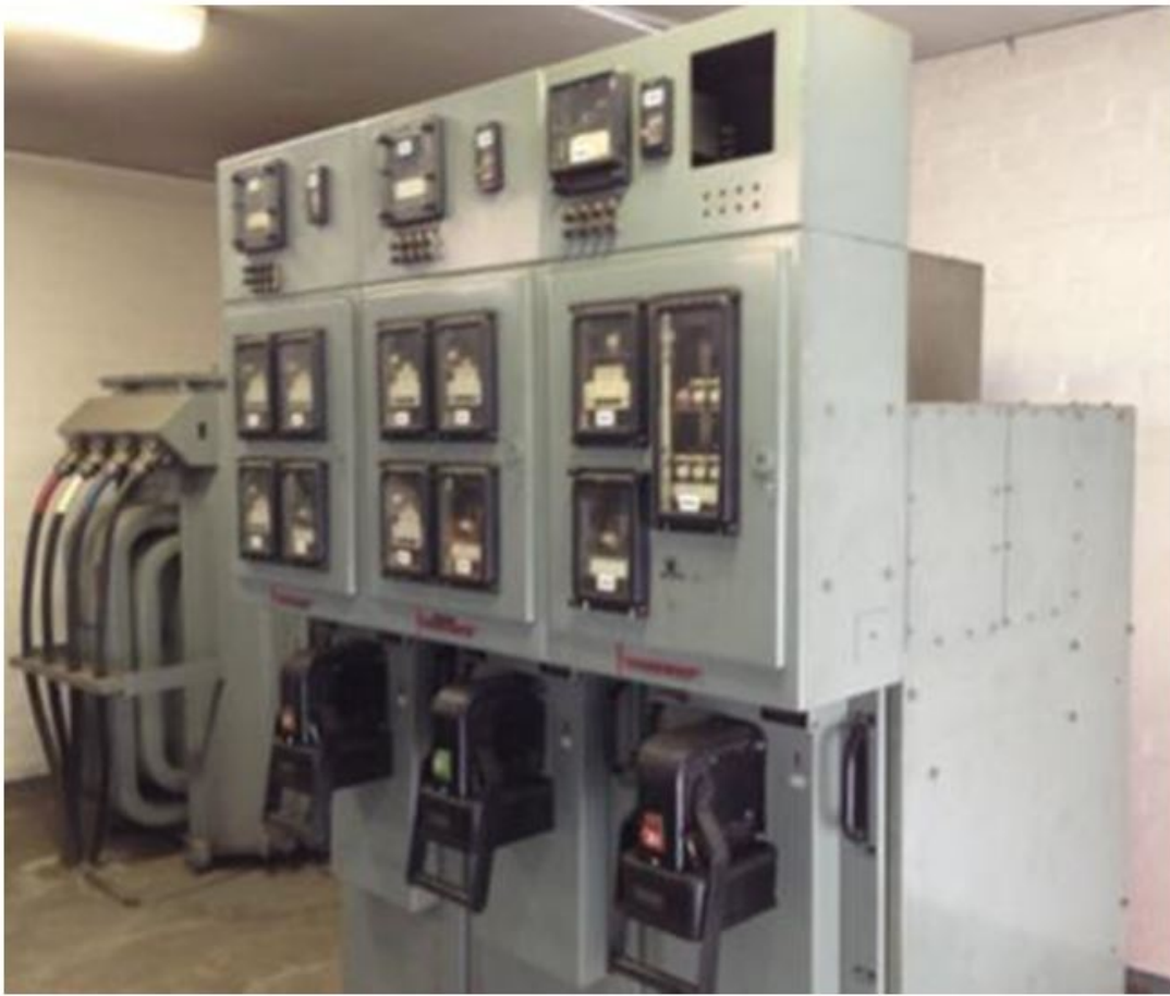
Figure 2 – English Electric oil filled switchgear.
