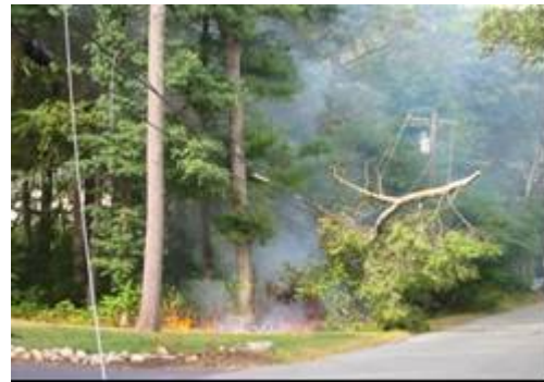
Photo 4: Multiple broken conductors
