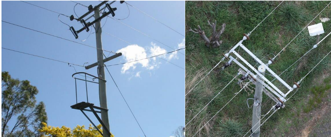
Figure 9: The same pole seen from the ground and from the air
