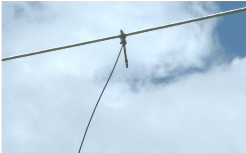
Figure 7: Live line clamp directly connected
