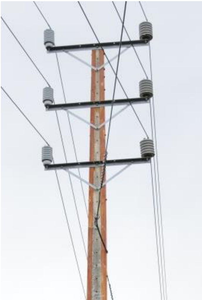
Figure 3: Steel HV crossarms
