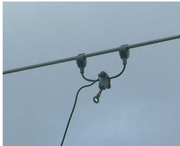
Figure 8: Live line clamp connected via D-clamp
