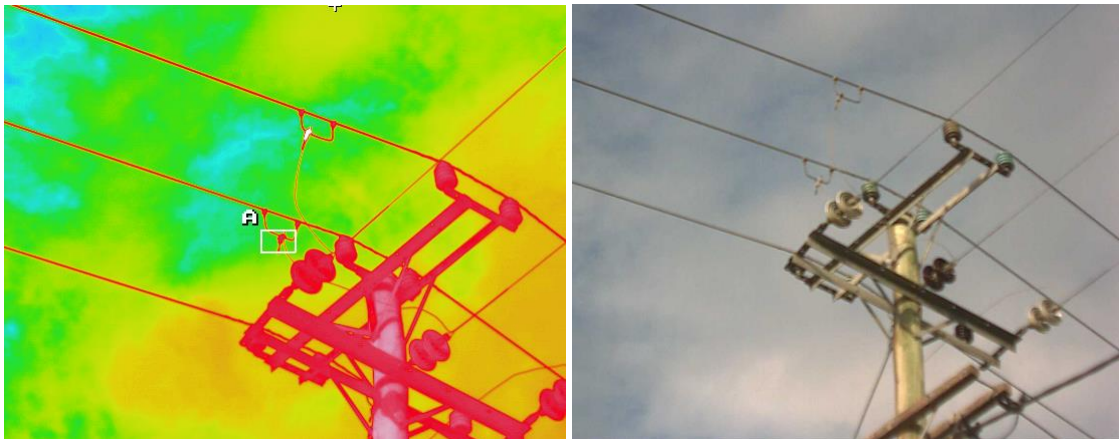
Figure 11: A Live Line Clamp through a thermal imaging camera and a normal camera
