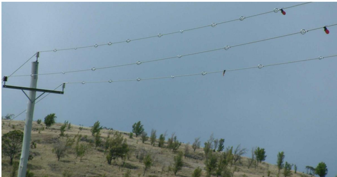
Figure 6: Bird diverters installed on conductor
