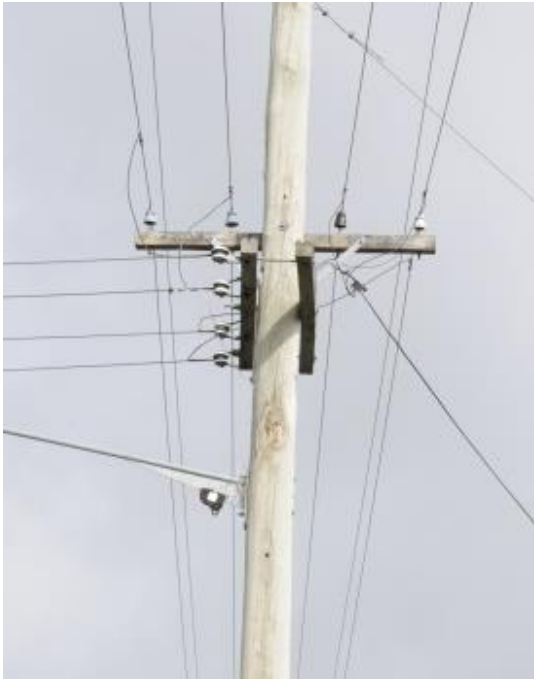
Figure 4: Wooden LV crossarms
