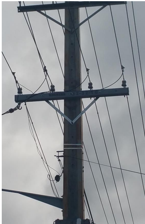
Figure 5: Fibreglass LV crossarm
