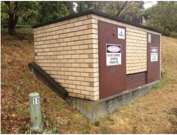
Figure 3 – Block wall kiosk (1977)
