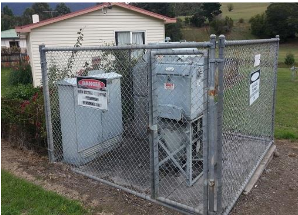
Figure 5 – Fence Type substation (1967)
