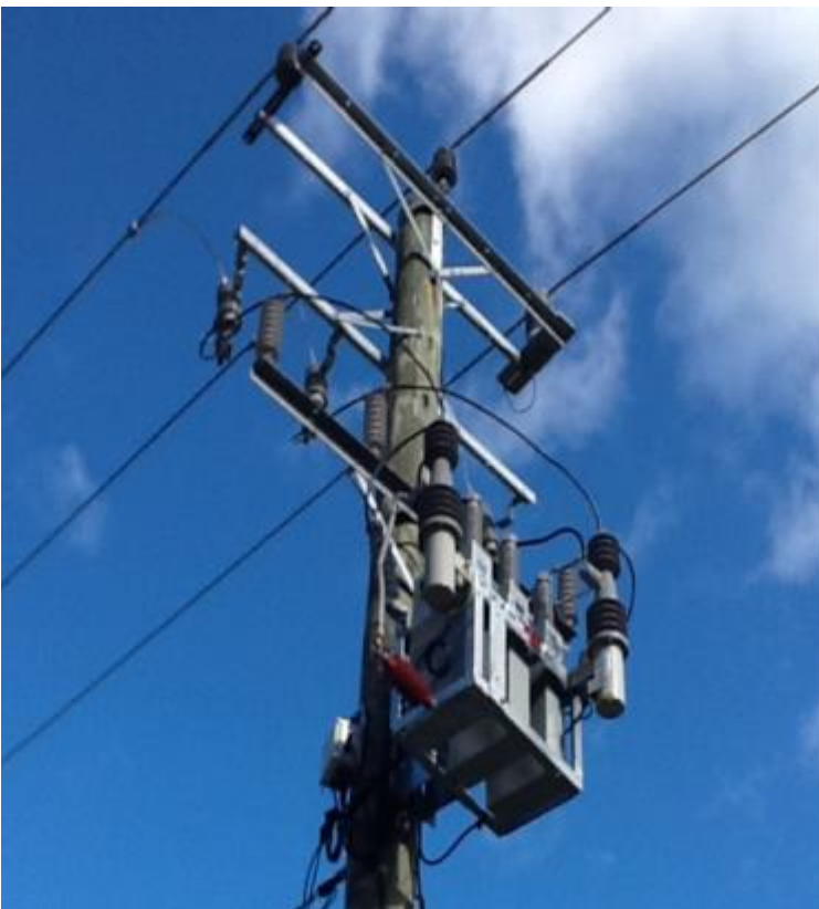
Figure 7: Pole mounted ABB capacitor bank
