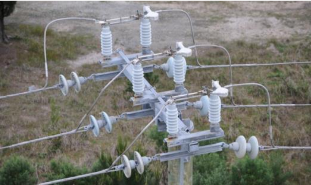
Figure 4: Horizontally operated air break switch
