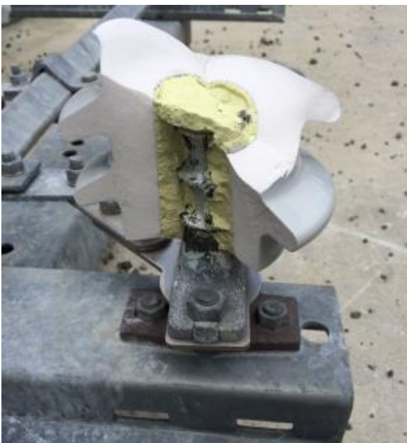
Figure 10: air break switch porcelain insulator pin failure
