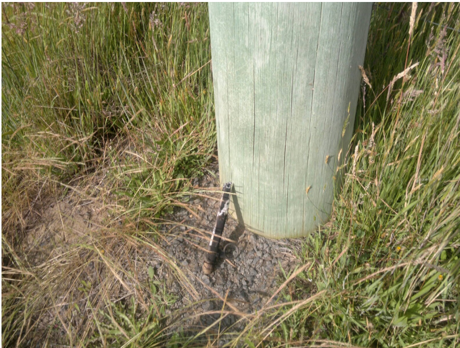
Figure 2. Failed EDO fuse tube
