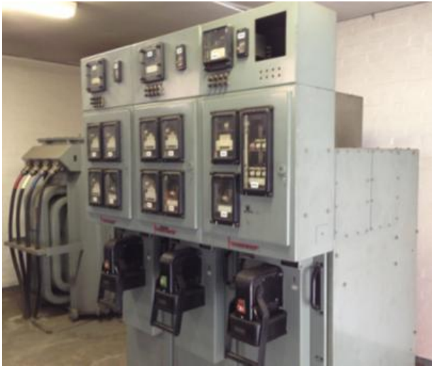
Figure 1 – English Electric oil filled switchgear.
