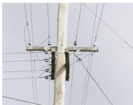
Figure 1: Sawn wooden LV crossarms
