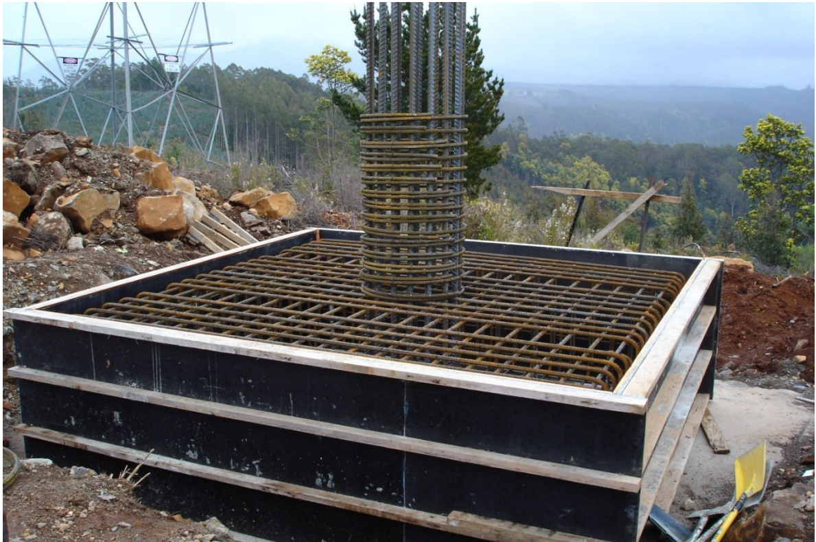
Figure 4: Example of reinforcing steel in concrete foundation
