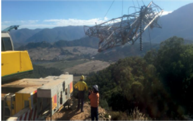
Steel tower affected by storms in southern NSW on 11 February 2017.
