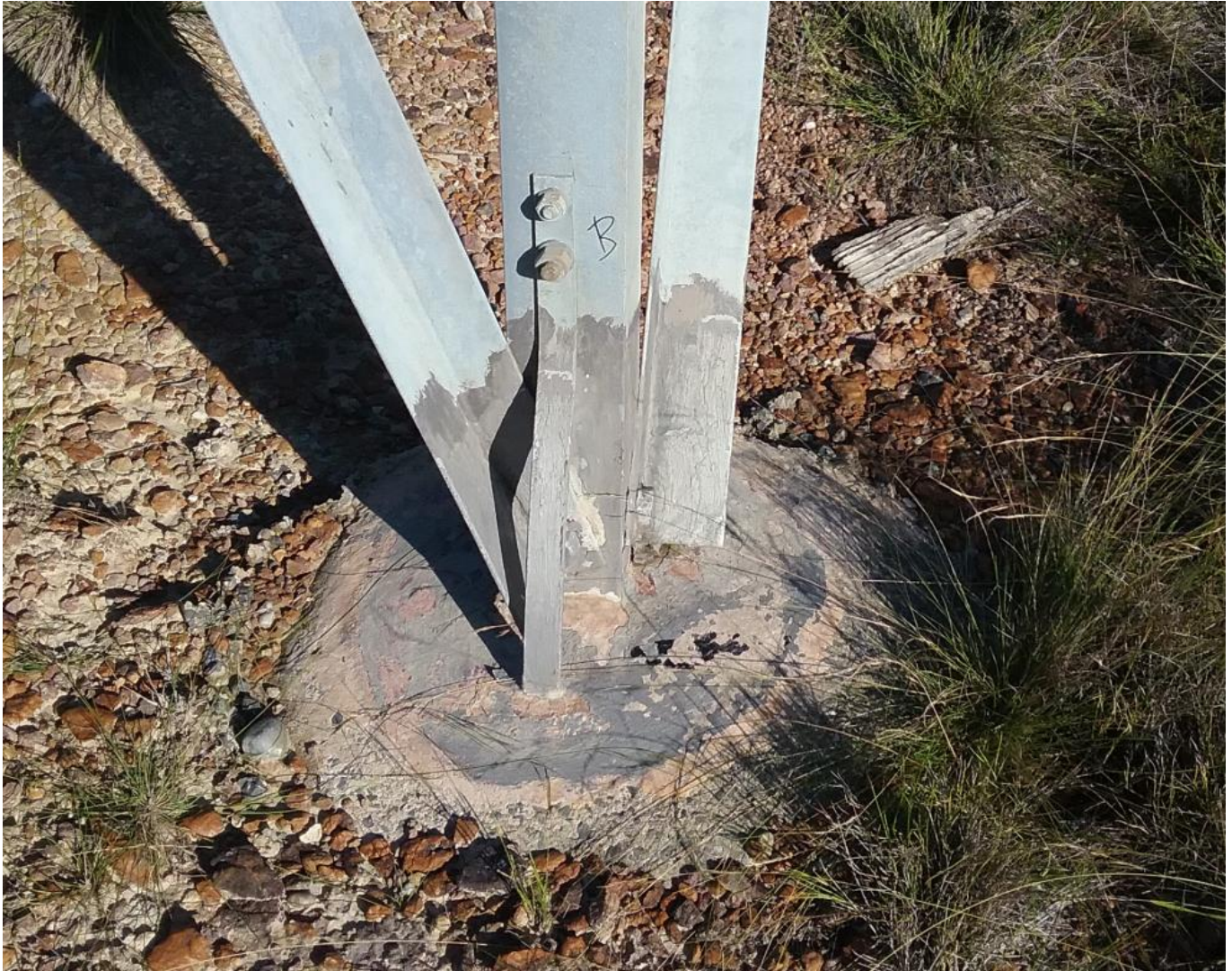
Figure 1 – Typical transmission line structure containing asbestos paint
