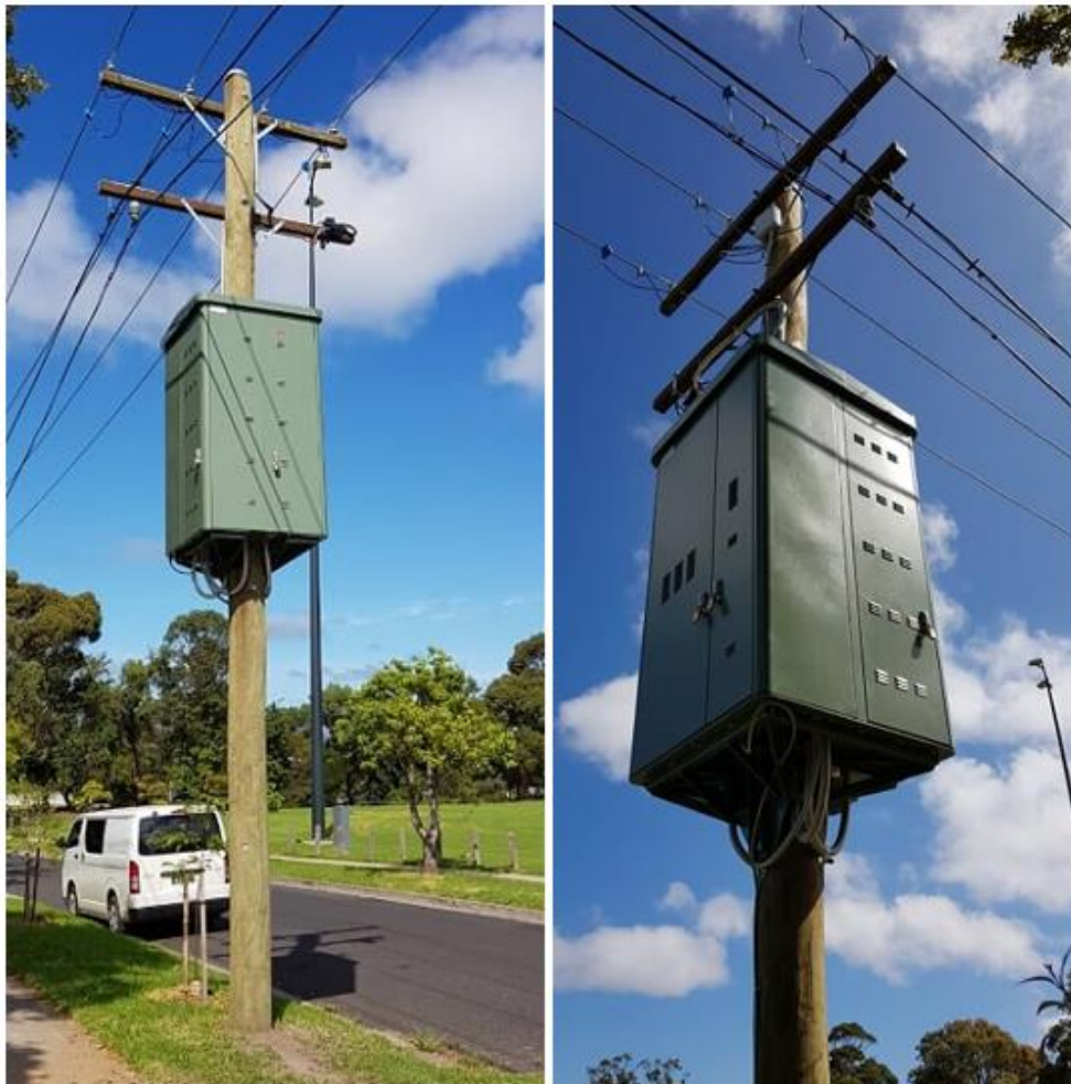
Figure 4: Installed BESS unit on UE LV network
