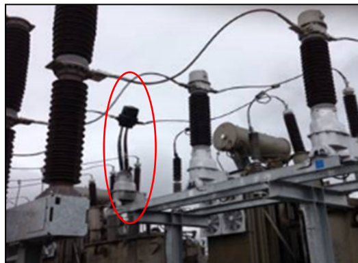
Figure 4| 132kV Current Transformer Explosive Failures
