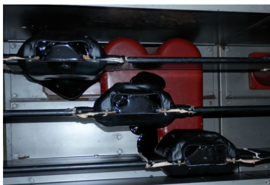
Figure 6| Old Pitch-Insulated Busbar Joints with Voids
