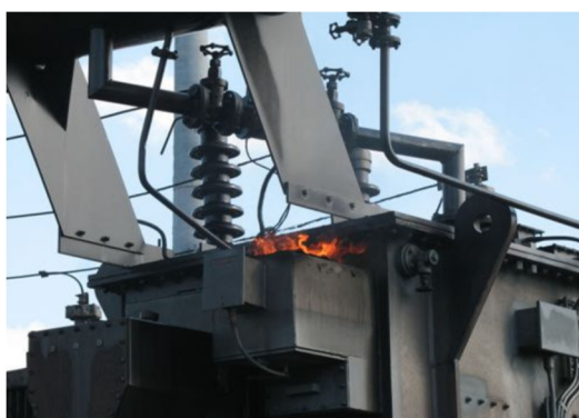
Figure 2| VT on Fire in Transformer Cable Box.
