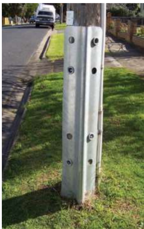
Figure 36: example of [REDACTED] RFD Pole Reinstatement 182
