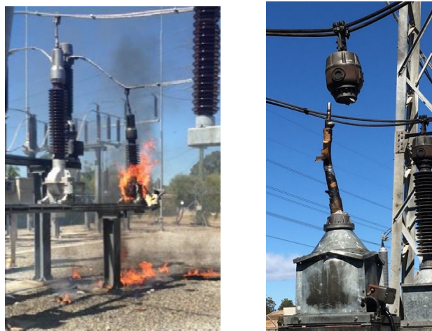
Figure 1| 132kV Voltage Transformer Failures (different substations)
