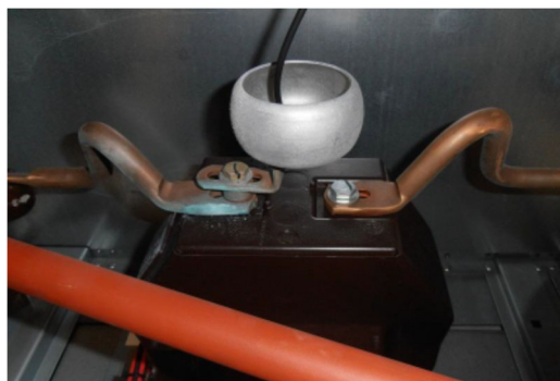
Figure 7| Contact Partial Discharge due to corrosion.
