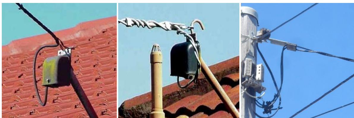
Figure 2.1 Sample images: neutral screen service, PVC grey twisted, and aerial bundled cables (respectively)
