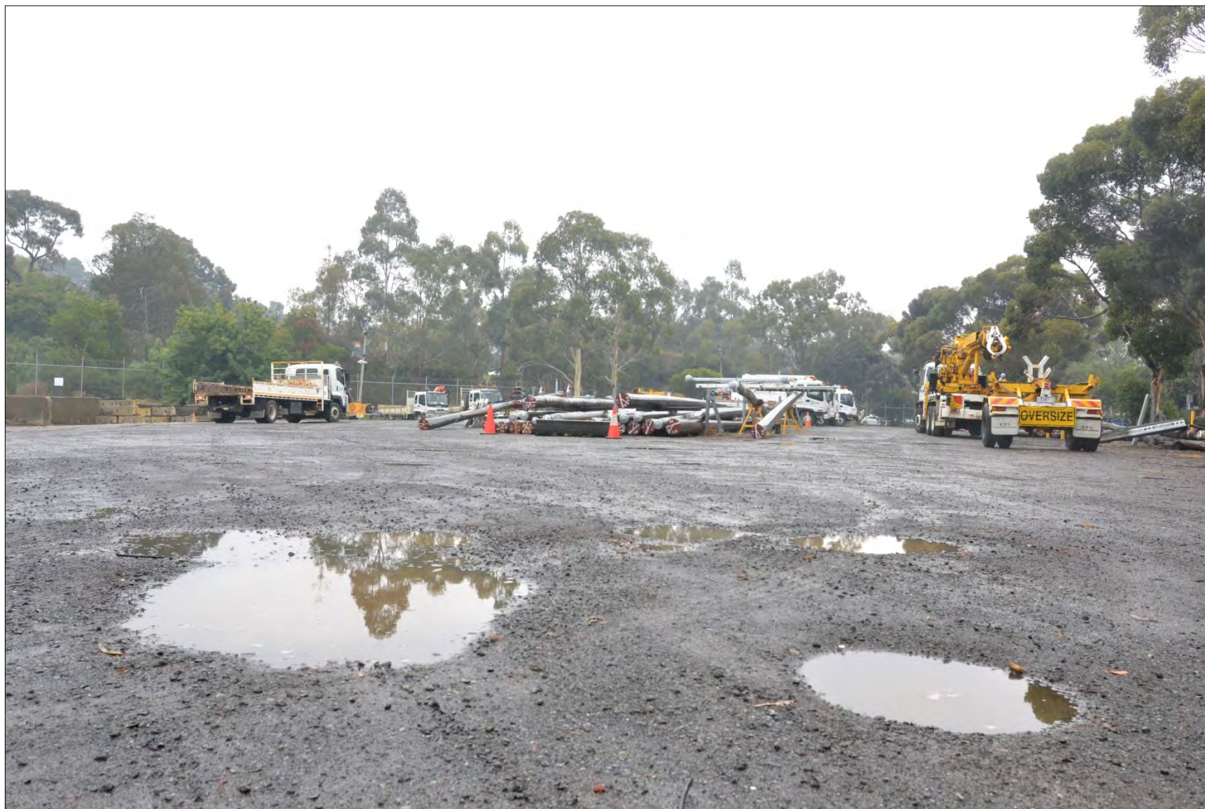
Figure 17: Improper surfacing, which causes vehicles to get bogged
