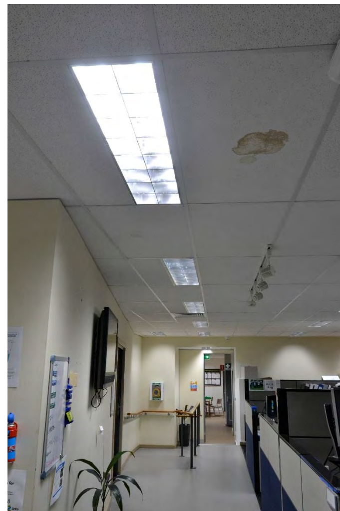
Figure 9: Ceiling further affected by leaks near light source
