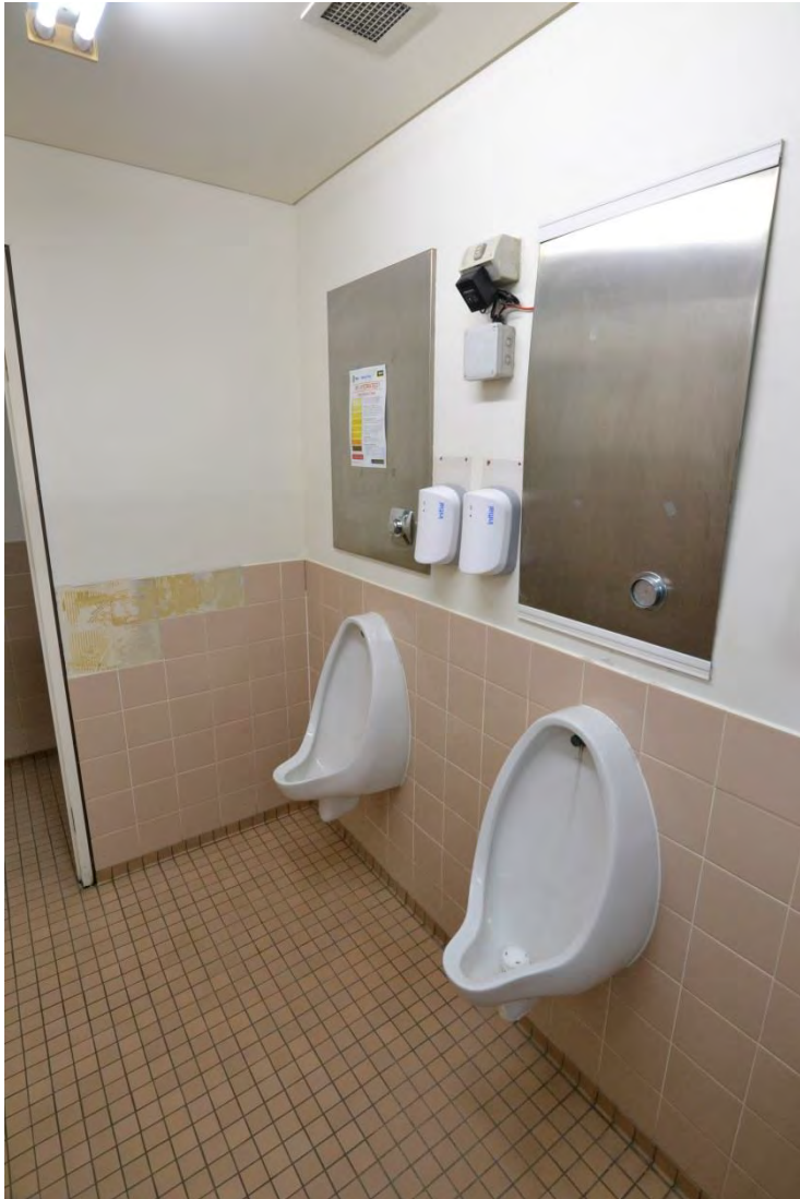
Figure 1: Male toilets with missing tiles
