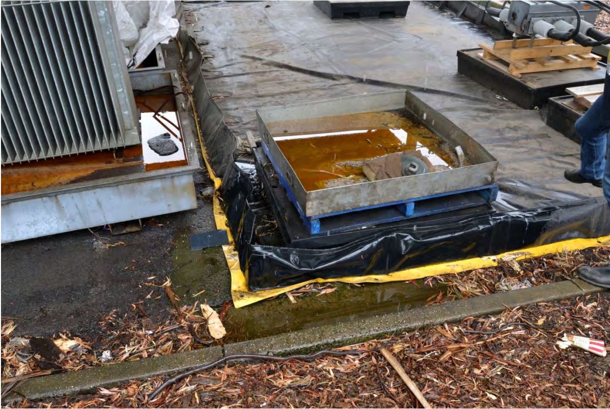
Figure 19: Inadequate and damaged bunding
