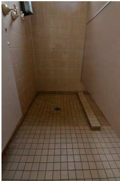
Figure 4: Male showers with steep floor gradient
