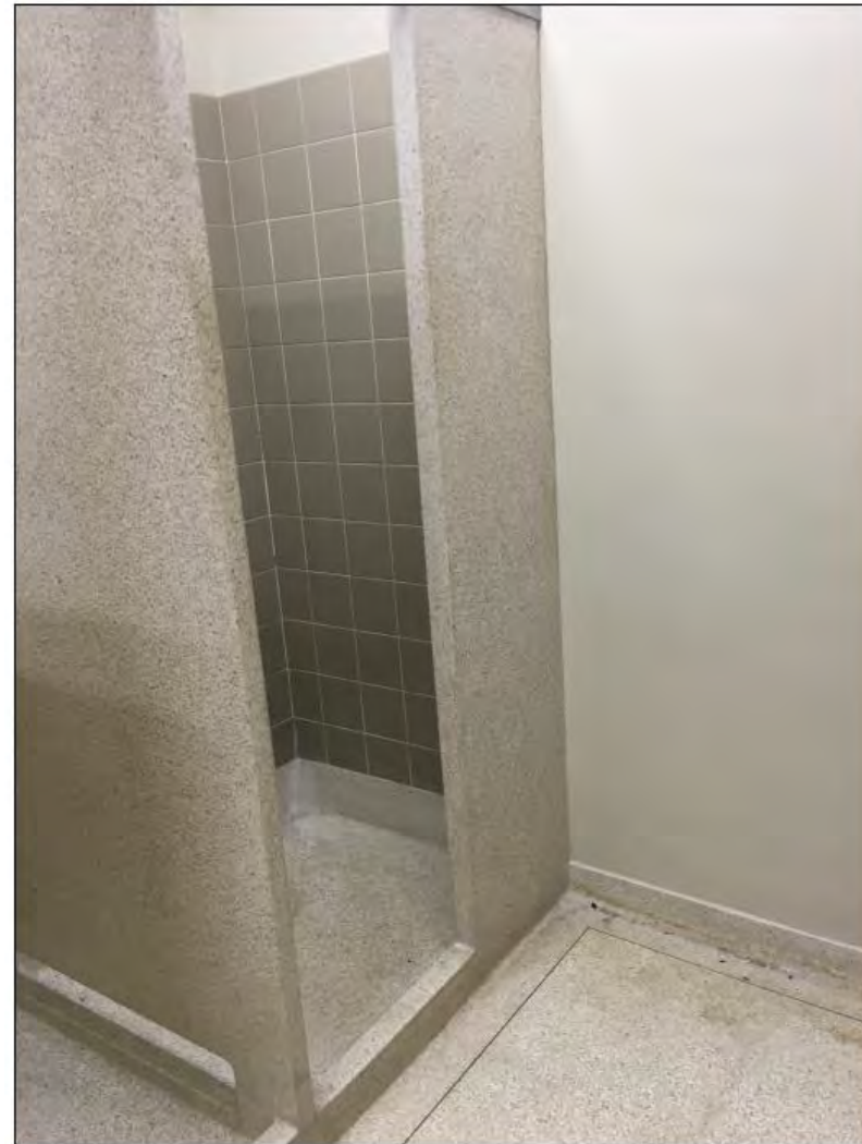
Figure 12: Showers with no privacy doors or curtains, high ground-edging and no slip rail
