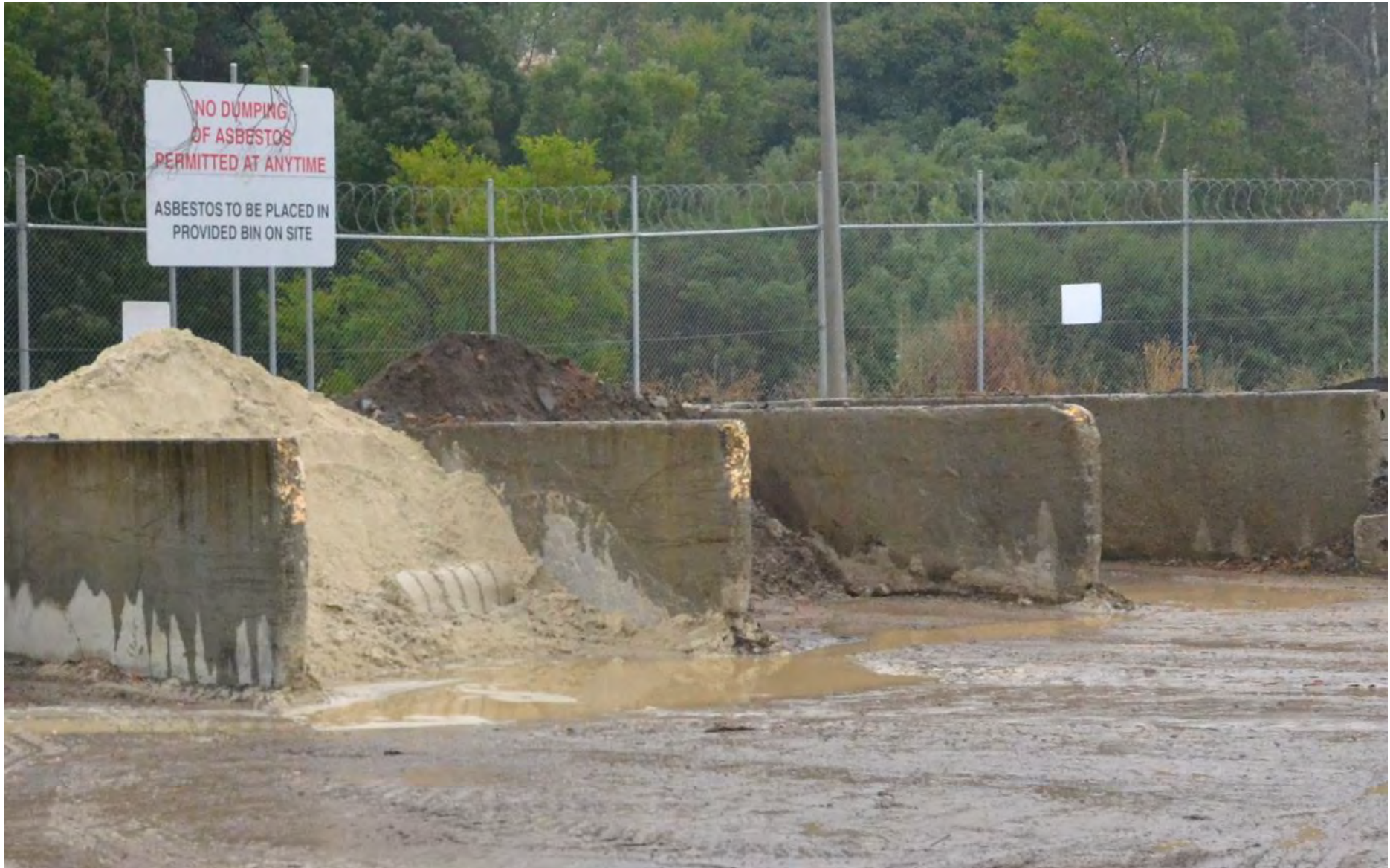
Figure 18: Improper surfacing, which causes vehicles to get bogged
