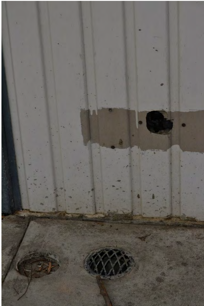
Figure 18: Hole in front exterior wall due to urgent repairs to flooding septic tank
