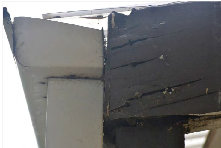
Figure 14: Enlargement of rot
