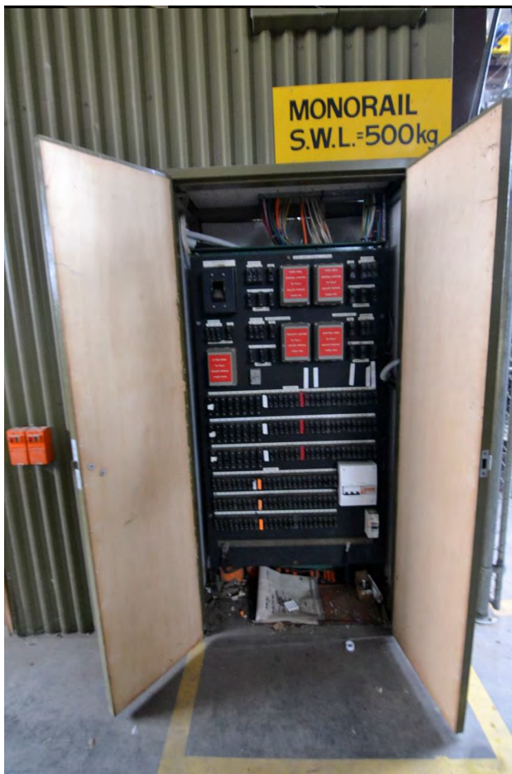
Figure 2: Old switchboard without blast-proof doors, exterior ventilation or other containment
