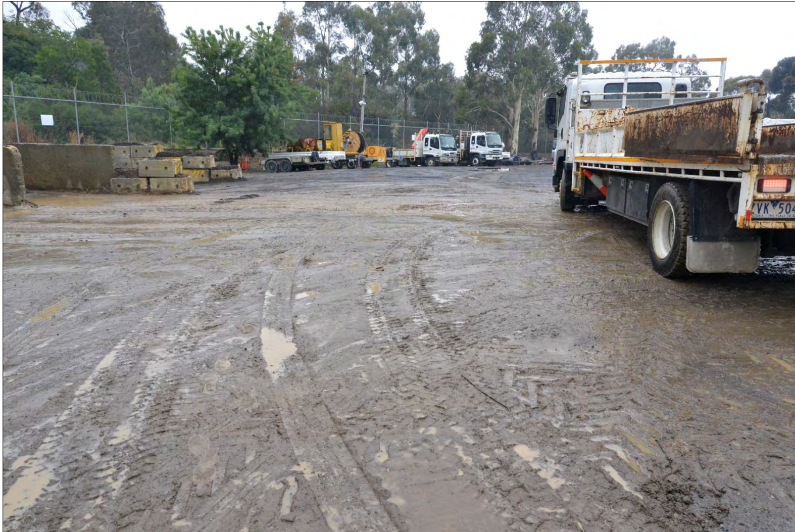
Figure 16: Improper surfacing, which causes vehicles to get bogged
