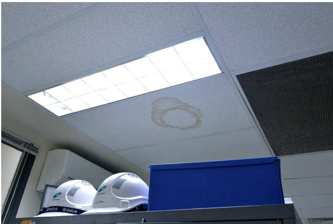
Figure 8: Ceiling affected by leaks near light source
