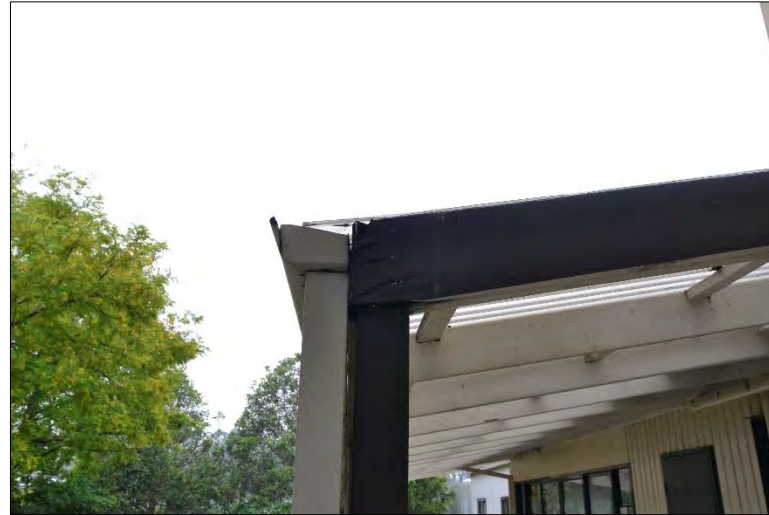
Figure 13: Rotting timber in end awning
