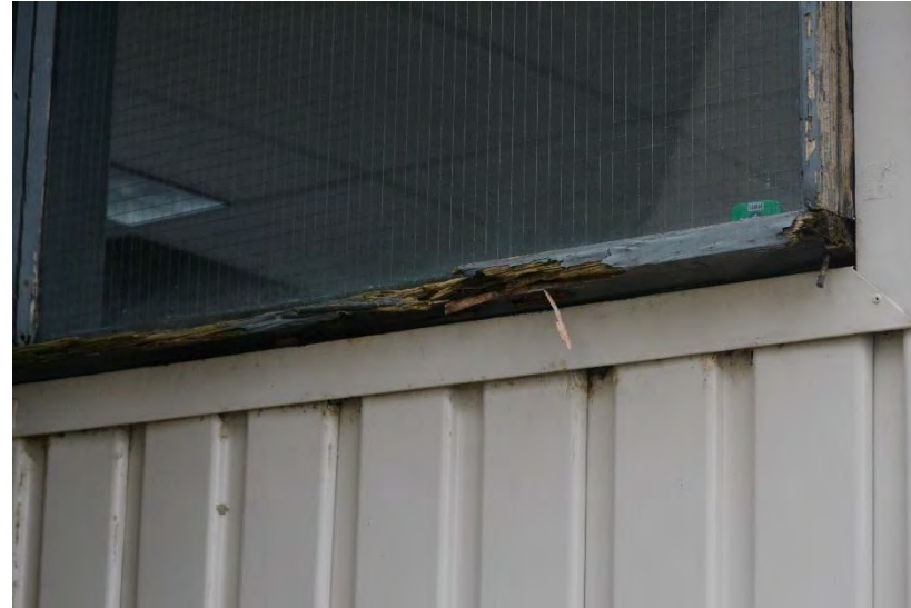
Figure 16: close up of rotting window
