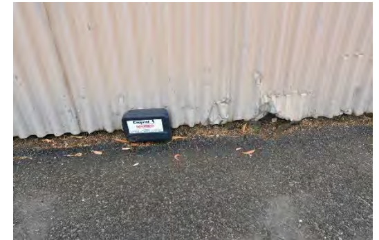
Figure 6: Damage to exterior of Building E and vermin control measures
