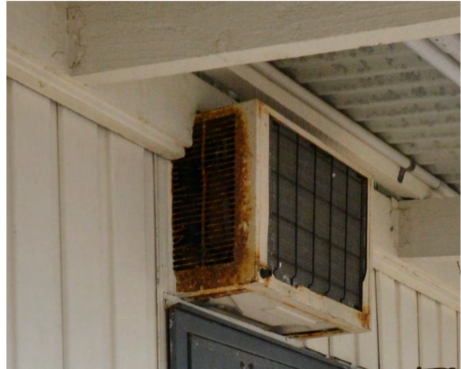
Figure 11: Close up of rusted air conditioner present in external walkway
