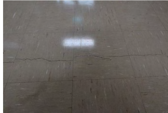
Figure 5: Cracked floor tiles
