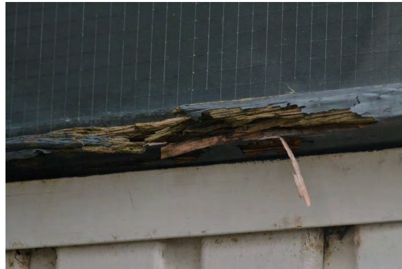
Figure 17: further enlargement of rot
