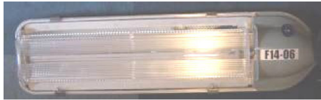
T5 twin 14W (Pierlite) low-energy light
